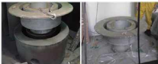
Separation of Graphite and Reflector Housing
