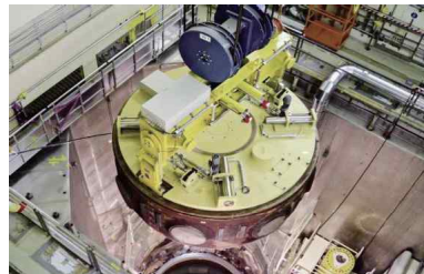
Lifting of Cut Ring
