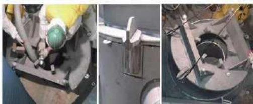
Removal the in and outside of Reflector Housing
