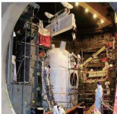
Lifting of steam generator from the cubicle.
